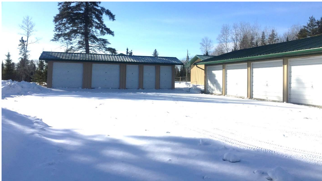
Photo 2 – View of the northeast side of the storage buildings
