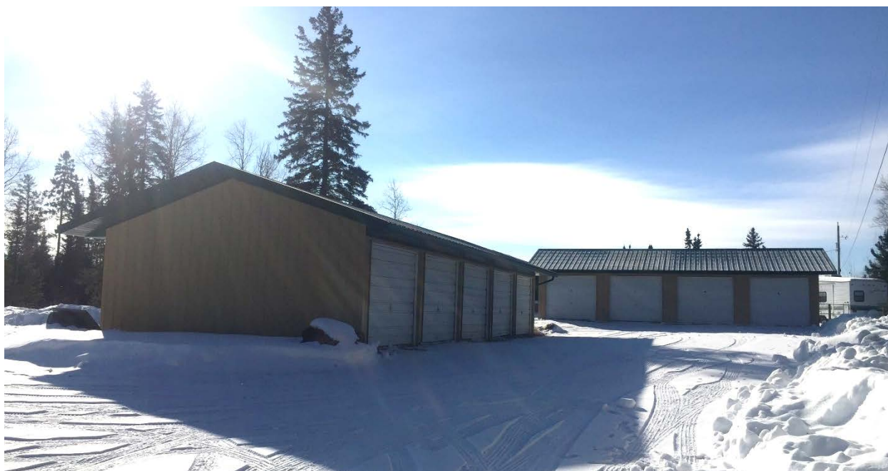
Photo 3 – View of the northwest facing side of the storage buildings
